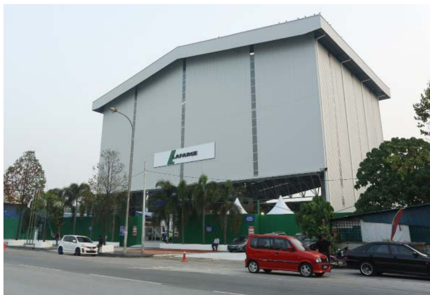
State-of-the-art enclosed ready-mixed batching plant in Chan Sow Lin, Kuala Lumpur, an industry benchmark for batching plants in urban cities.
