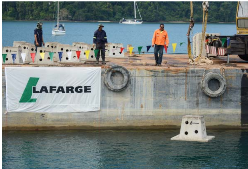
A full-scale deployment of the Artificial Reef Module System (ARMS) in the vicinity of Datai Bay, Langkawi.
