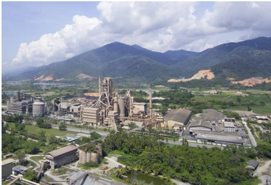
Our Lafarge Kanthan Plant has contributed significantly to the development of Perak for over 50 years.
