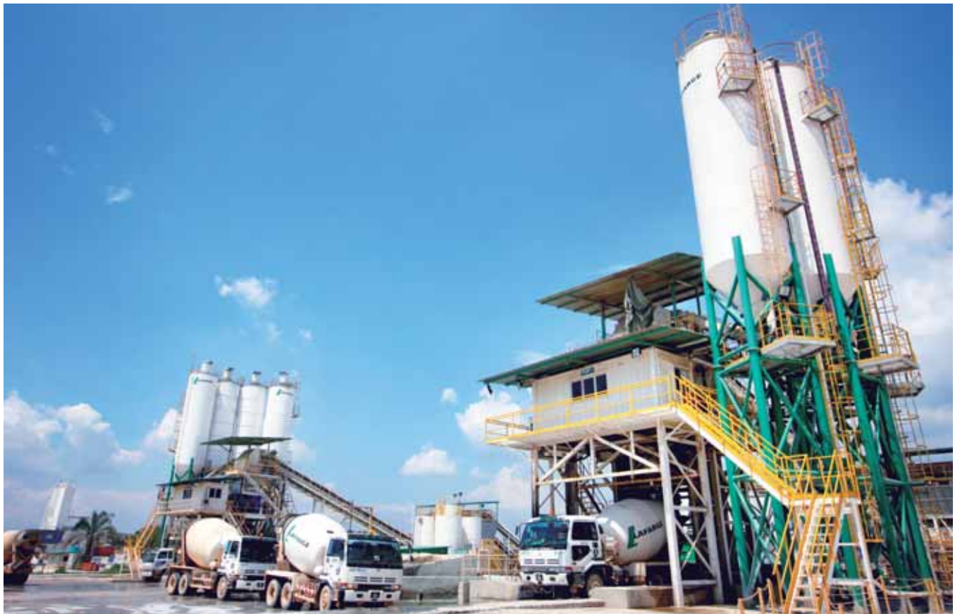
One of Lafarge Malaysia's ready-mixed concrete batching plants.
