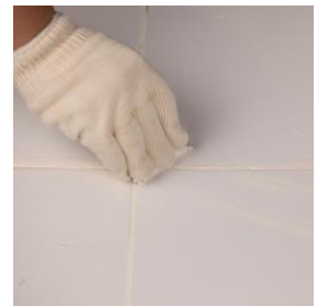
Application step 2: Remove excess tile grout
