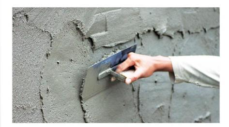
WALLCEM is a masonry cement specially formulated by intergrinding portland cement clinker with plasticizing materials and air entrainment agent to achieve a high fineness and good workability for plastering application. It is suitable for internal and external plastering works.
